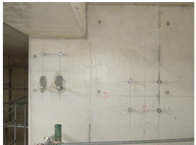
<M16 新型偏心地脚螺栓施工完毕>
