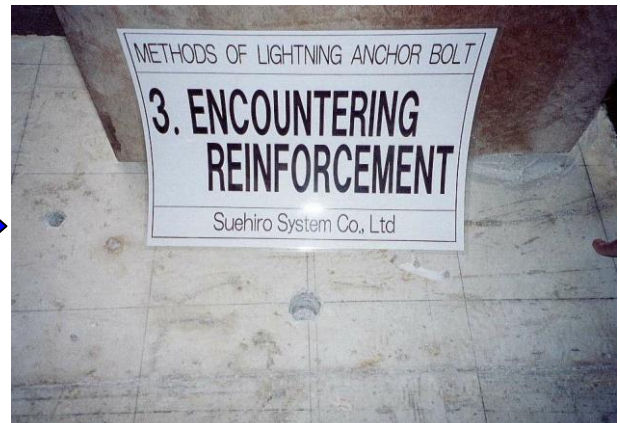
<Re-bar at drilling position>
