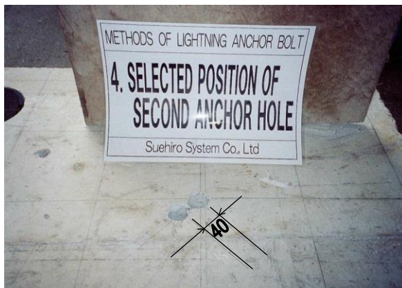
<Drilling of 2nd anchor bolt hole>
