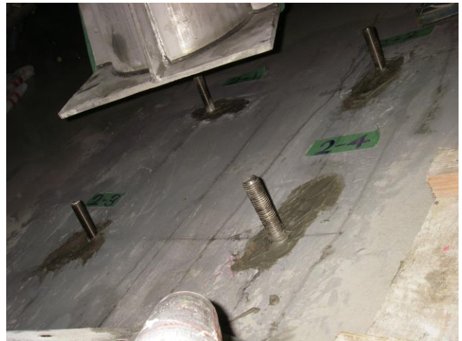
<Installation of Deflective Anchor Bolt>
