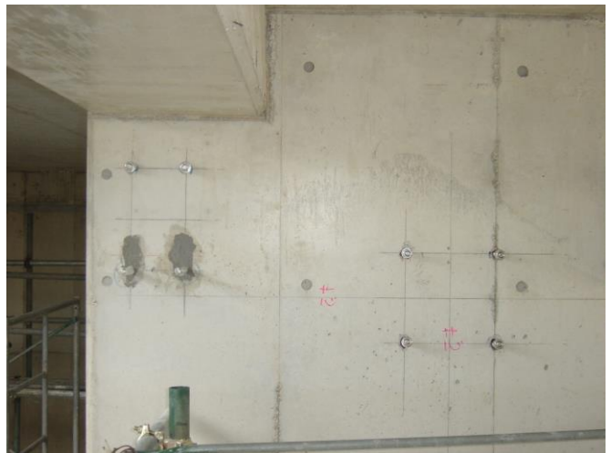
<Completion of M16 new-type Deflective Anchor Bolt installation>
