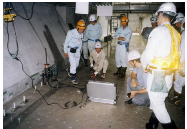
<Anchor pull-out test>
