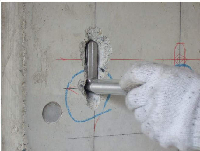
<Temporary insertion of M16 new-type Deflective Anchor Bolt> Example of test 5)
