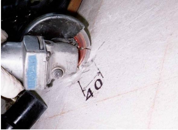
<Cutting the concrete surface with a cutter>
