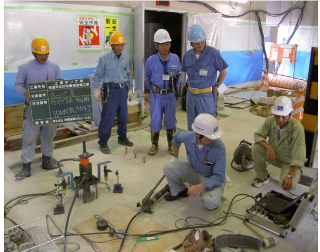
<Anchor pull-out test>
