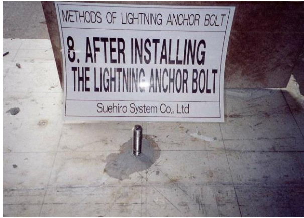
<Completion of Deflective Anchor Bolt installation>
